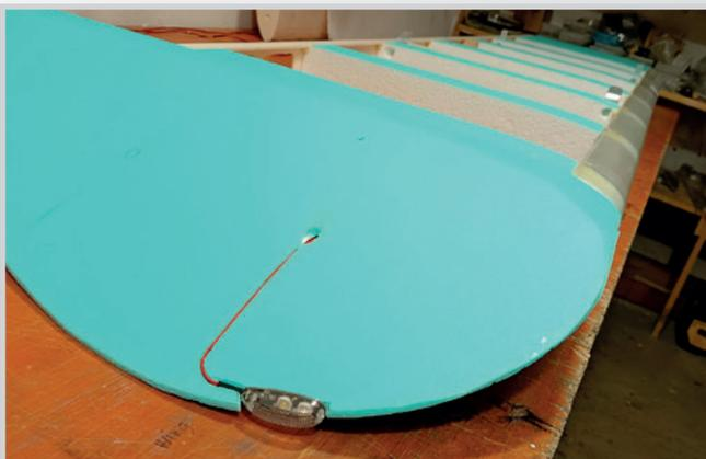
cover rudder with light balsa 1,5 mm
